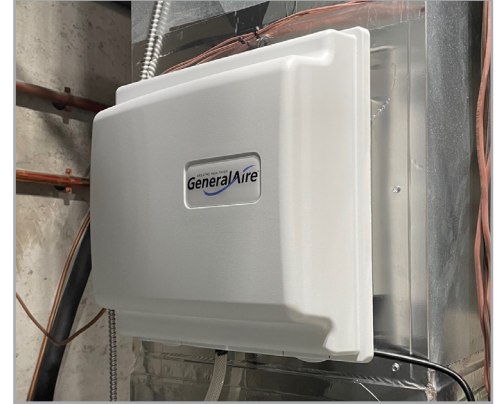
Vertical Supply Plenum Installation Only
