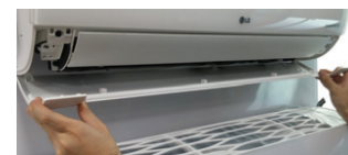
Figure 104: Checking that All Attachment Locations Are Secure (Step 5).
